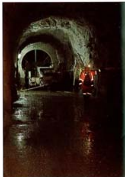
Tunnelling the 5m-diameter headrace.
